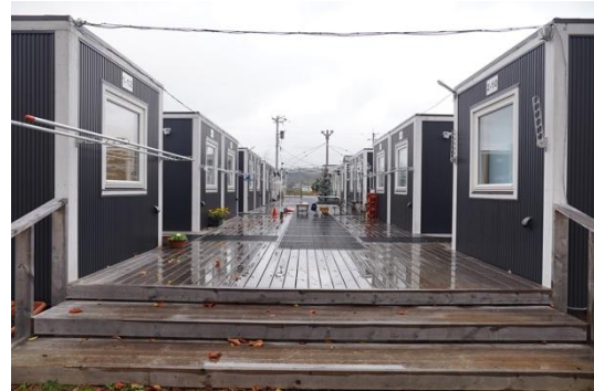
Figure 2. Container-Type Units Deployed in Shika Town
